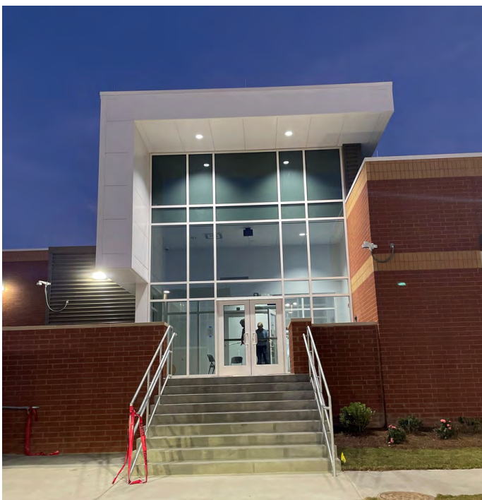
Charleston Juvenile Detention Center - under construction 12/2021
